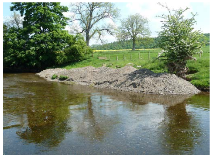
Figure 5: Dredging of the River Lowther
