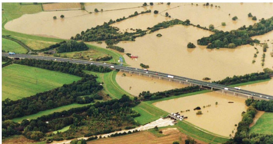
← Flood water storage at the Leigh Barrier.
