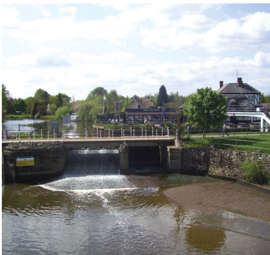
Weir system from Twyford Bridge on the → River Medway, Yalding.
