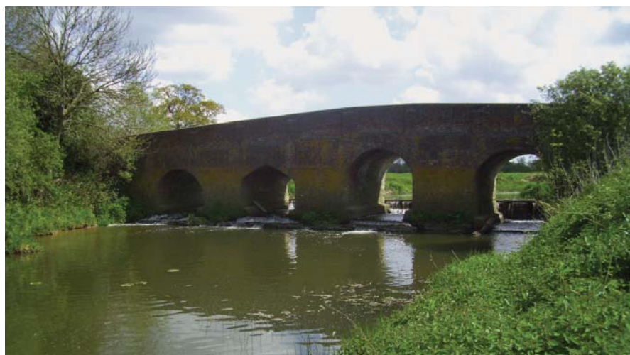
←Hawkenbury Bridge over the River Beult, near Staplehurst.
