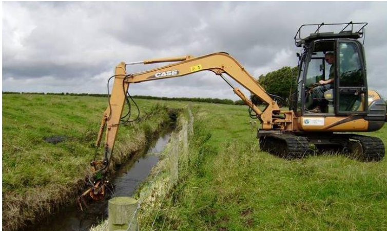
Figure 4: Use an appropriate sized machine and bucket
