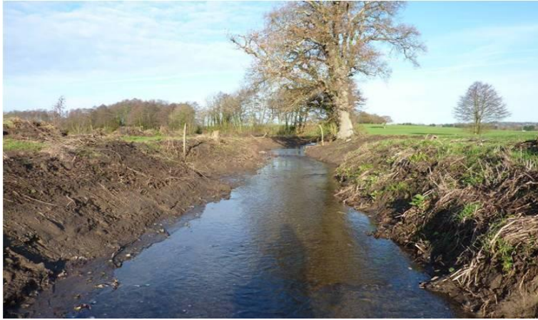
Figure 6: You should not leave banks bare or exposed after de-silting
